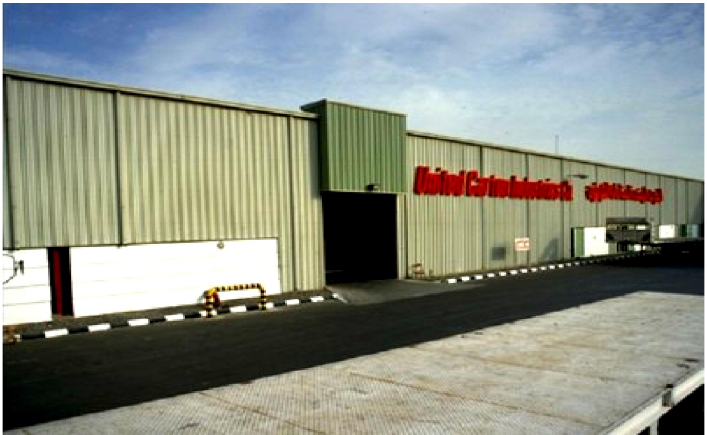
United Carton Factory-Jeddah
