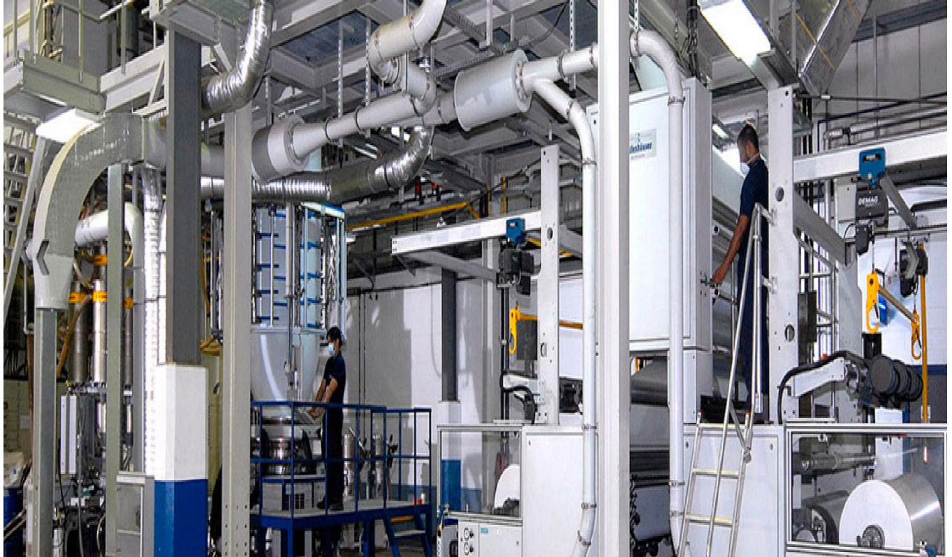
Al Tayar Plastic Factory-Jeddah
