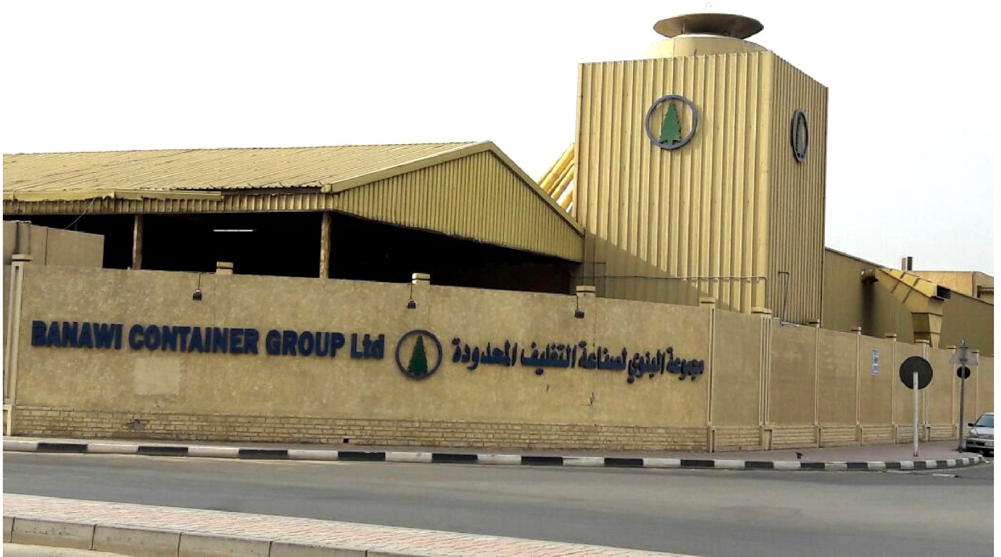
Banawi Corrugated Packaging Plant-Jeddah
